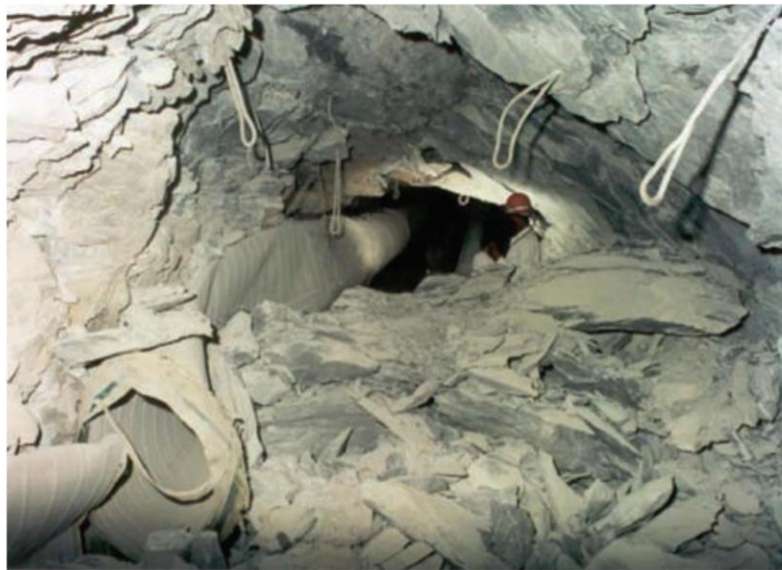
Figure 1 Aftermath of a rockburst in a deep-level mine (Photo W.D. Ortlepp)
